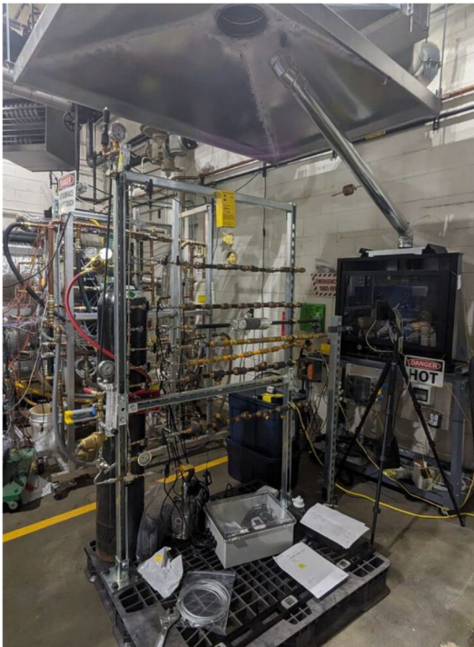
Leakage test apparatus during shakedown tests.
