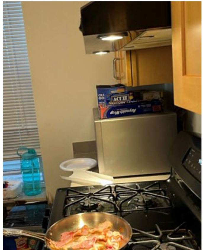
Frying Bacon and Eggs on a Gas Range Top in the ENERGY STAR Residential Unit with a Direct Vent Range Hood
