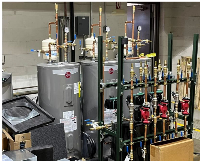
Test stand construction starting in May 2024
