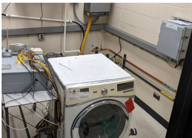
New Environmental Test Chamber during Construction
