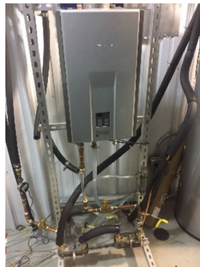
LG 25MBH heat pump with evaporator outside (left), tankless water heater with condenser heat exchanger (middle), condenser plate heat exchanger (right)
