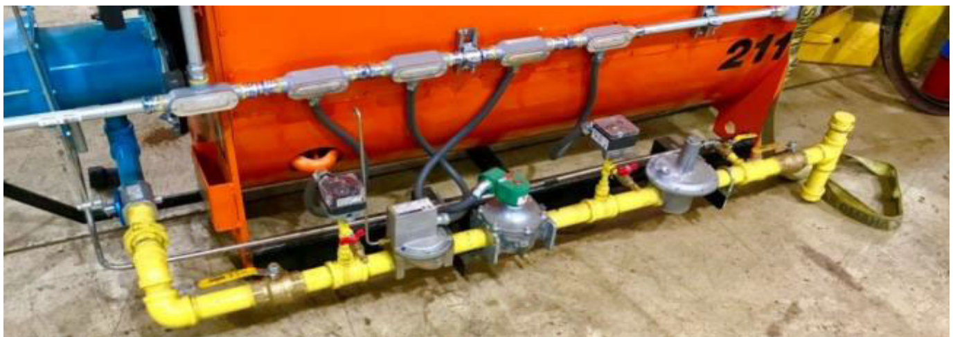
Example Boiler Gas Train (credit: Dungs)
