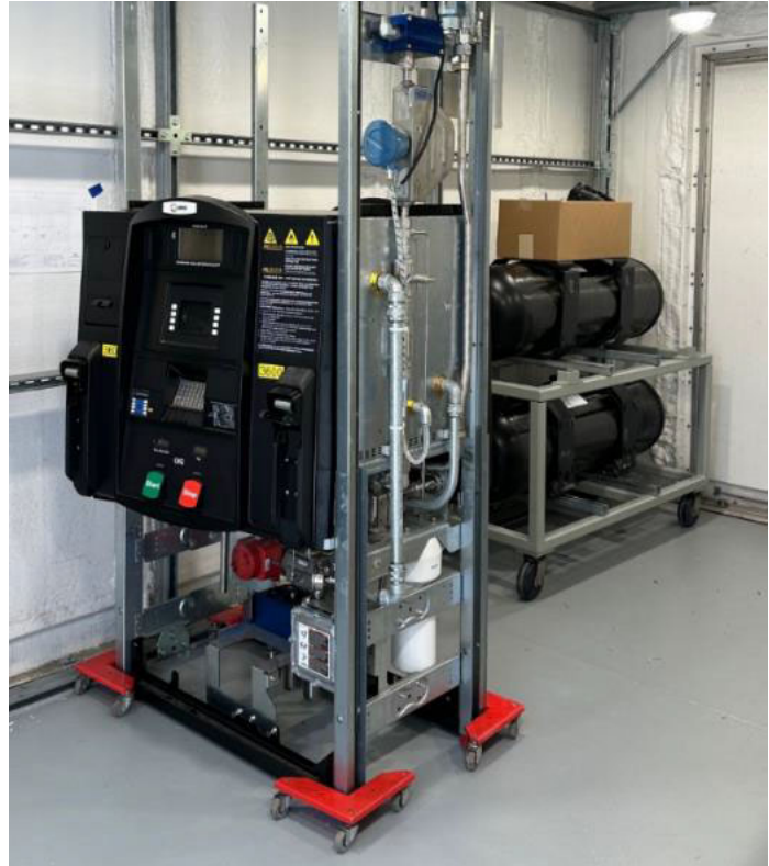
The ANGI dispenser in the test chamber along with two target cylinders. The Smart Controller is connected to the ANGI Modbus to monitor data coming from the dispenser. In parallel, it also receives data from the dispensers that is transmitted over Wi-Fi using HEM data collection hardware.
