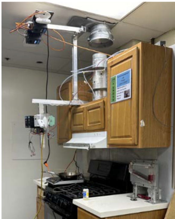
Residential Kitchen Ventilation Test Setup
