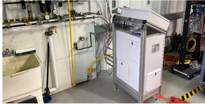
H2 Source and Mixer Undergoing Installation
