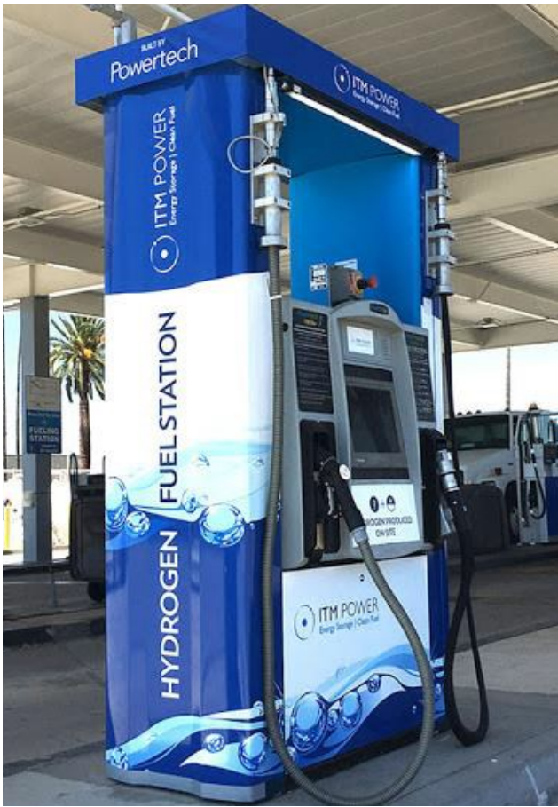
Hydrogen fueling dispenser. Image credit: California Energy Commission
