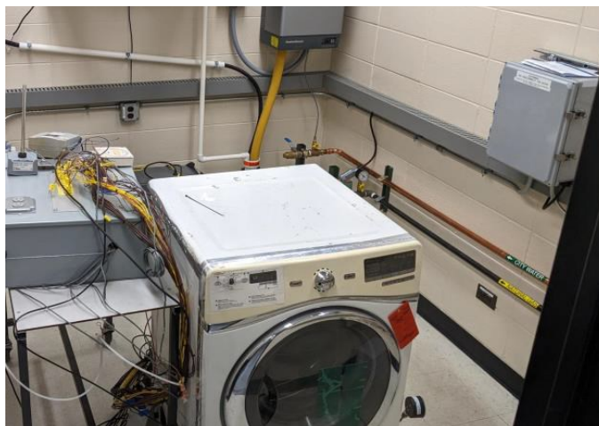
New Environmental Test Chamber during Construction
