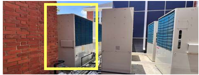
One of seven two-pipe GHPs installed at Pike Road School in Alabama.
