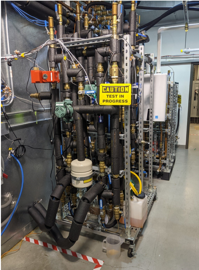
Completed laboratory test stand.
