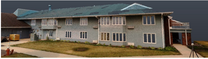
Point cloud image result from lidar scan of multi-family building
