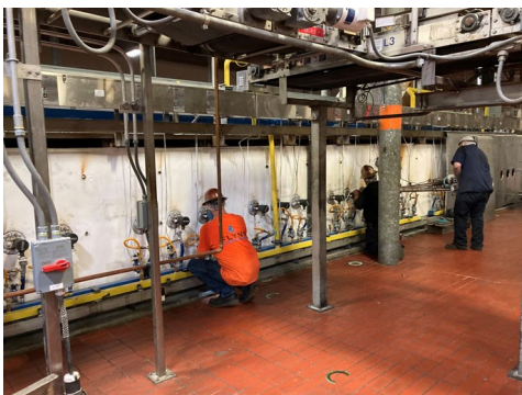
Combi-burners, zone 5 replacement and interior re-firing
