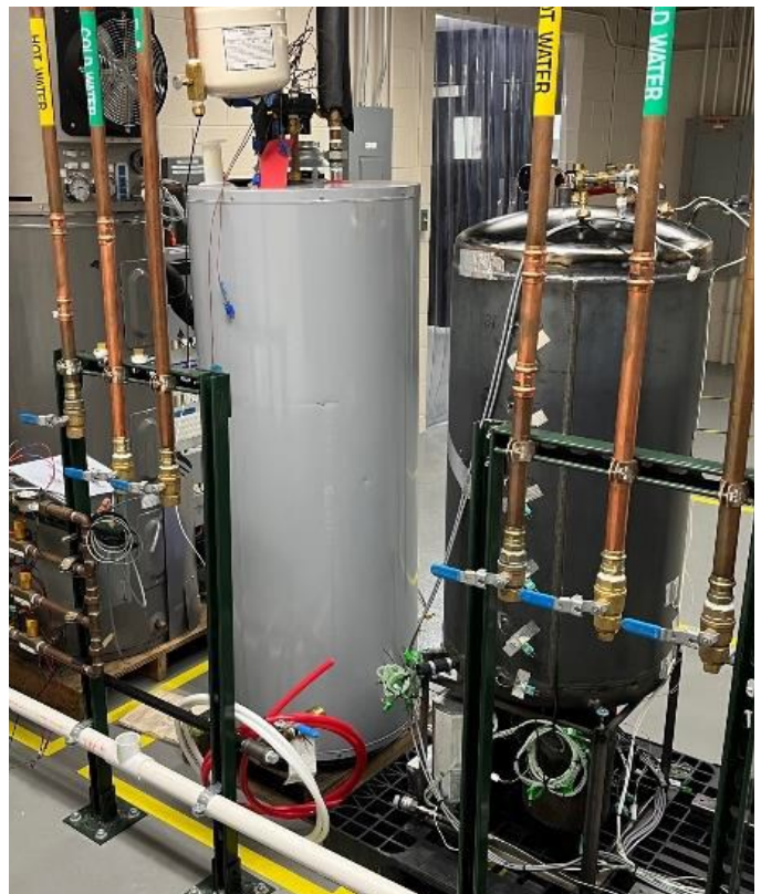
Water Heater Testing Area Test Installation Progress
